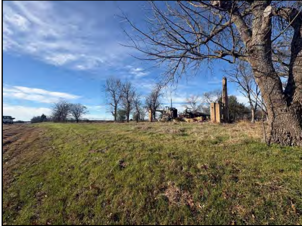
Photo 9. A burnt down house adjoining the subject property, facing west.
