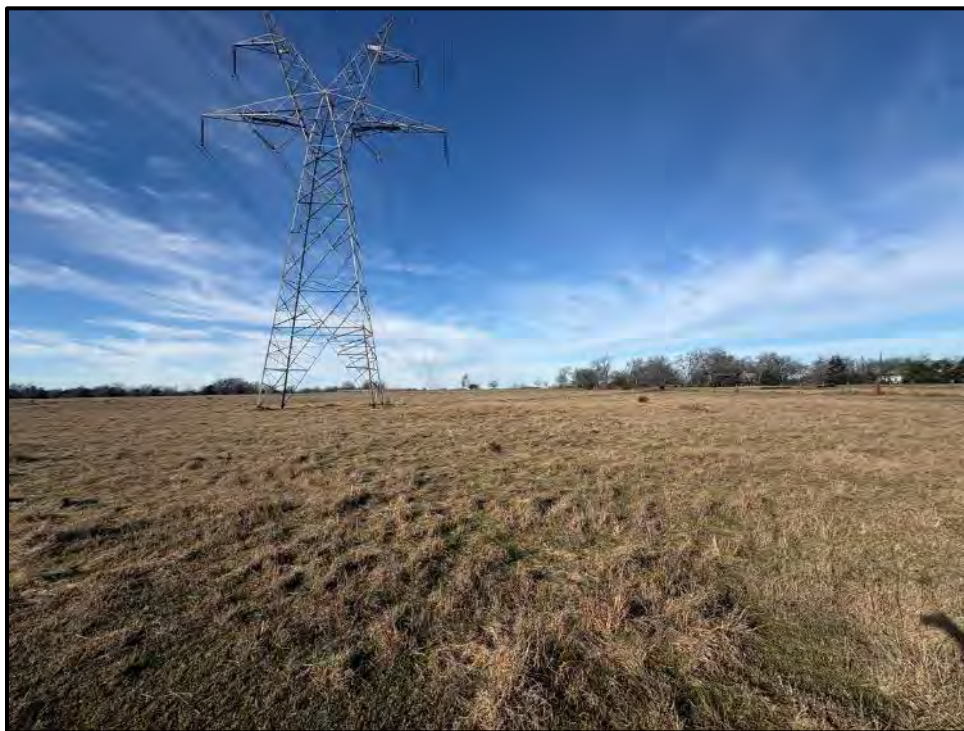
Photo 4. Electrical transmission line that traverses the southern portion of the subject property, facing west.
